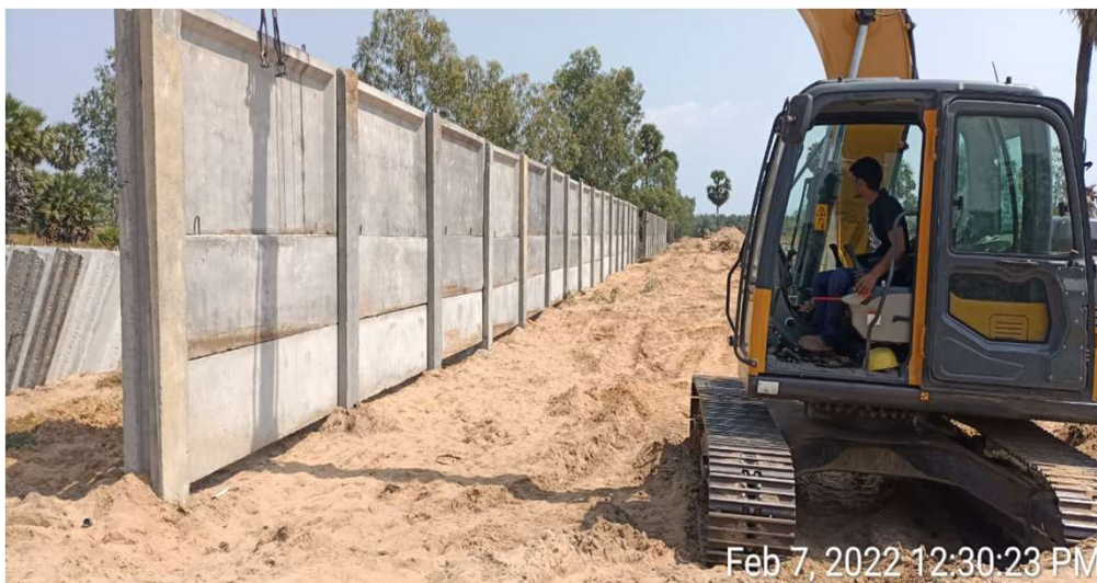
Adani Port – ABAN PLOT Compound wall
