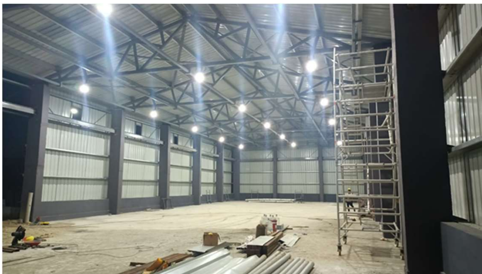
Adani Port – CFS Warehouse
